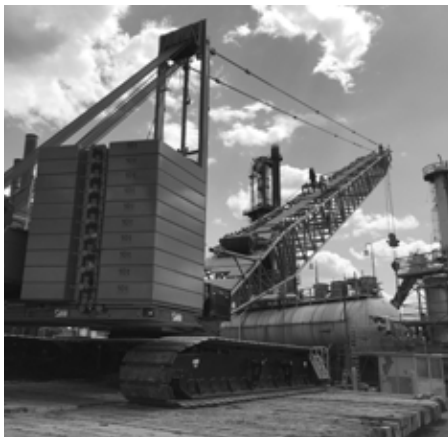
A crane secures a vessel that had been leaning due to the fire.
